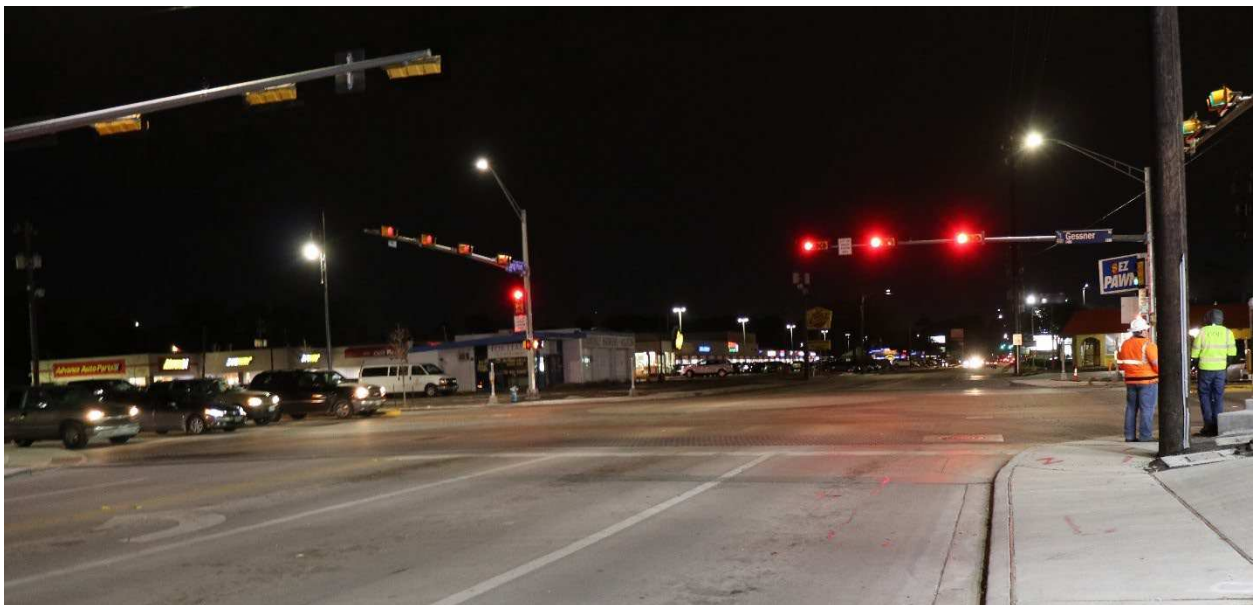
Figure 4: Lighting and missing crosswalks.
